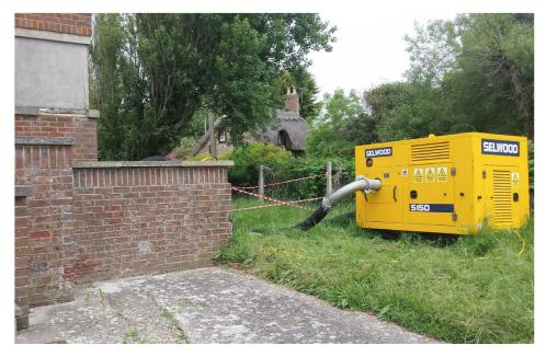
suction point. It was decided to utilise the power supply from the broken pump and connect an electric S150 Super Silent in place.
